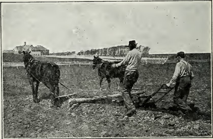
Fig. 61. Filling the ditch with a plow.
