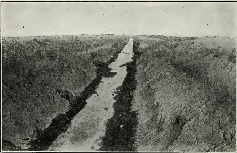
Fig. 43. An open drain.
