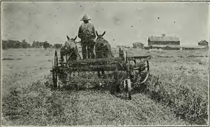
Fig. 166. A three-bar side-delivery rake at work.
