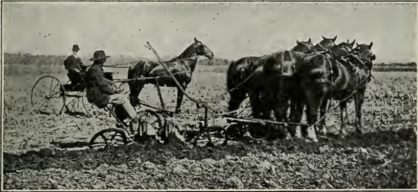
Fig. 115. A modern disk gang plow at work.
