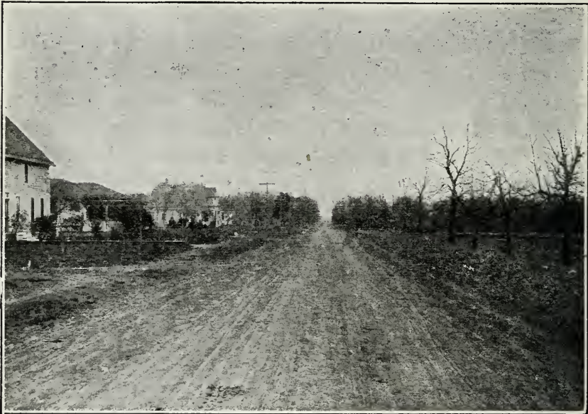
Fig. 80. An earth road maintained in good condition by the road drag.
